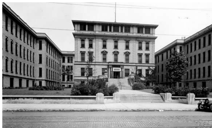
The building that is now Abell Administration Center, flanked by the other wings of the old Louisville General Hospital, 1923.
